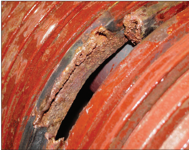
Figure 2. Conventional coil winding failure after improper repair.
